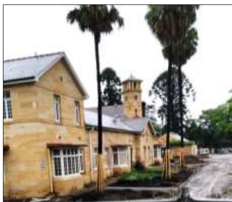
work has begun on new paving and garden beds!
