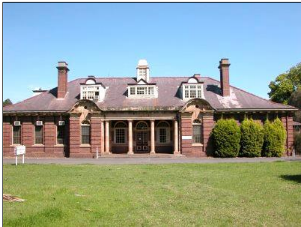
Liberty Vernon Building - site of Female Factory Gate entrance
