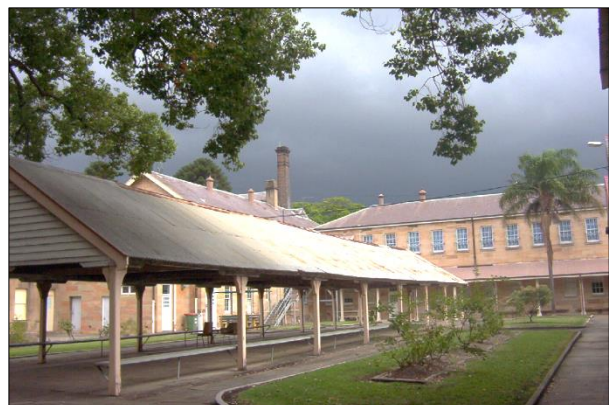
View of the Airing Yard (Female Factory period) with c1860 Pavilion
